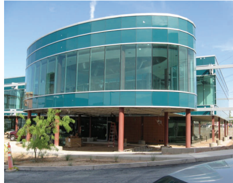
The DEC building during construction – 6/25/08
