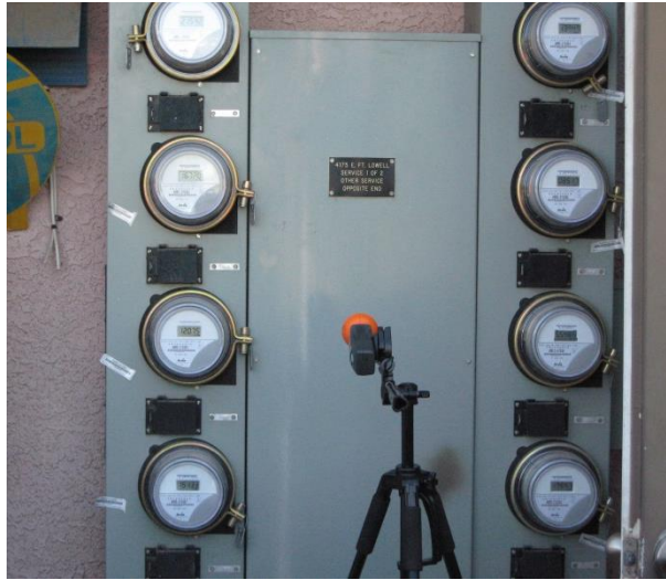
Figure 3. TM-195 placement at a bank of meters.
