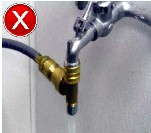
Figure 6—Unapproved Connection
