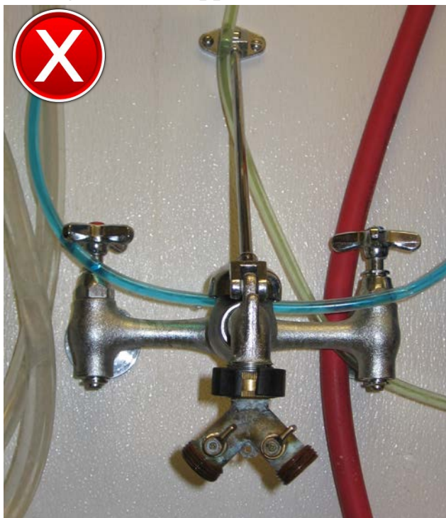
Figure 5—Unapproved Connection
