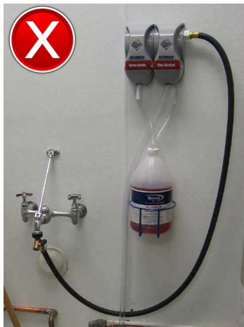
Figure 4—Unapproved Connection
