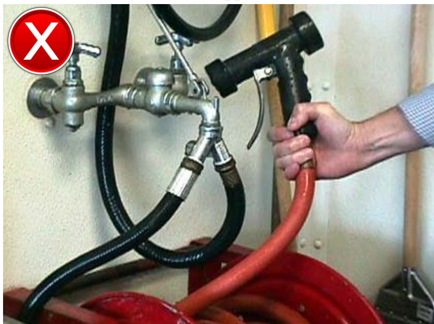
Figure 7—Unapproved Connection
