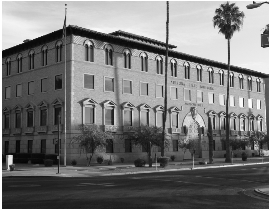
The Arizona State Building – 1688 W. Adams Street
